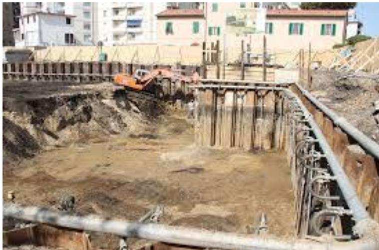
Figura 3-2: Sistema well-point abbinato a palancole
